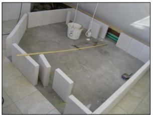
The adult enclosures were built of gaseous concrete (Ytong) blocks, glued to the concrete floor. Ytong blocks have little weight and are easily processed.
