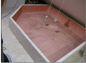
Subsequently, the rest of the floor and the Ytong blocks were coated.
