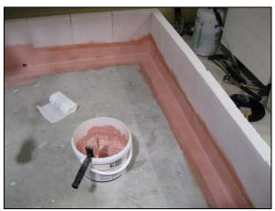
The corners were coated to ensure water tightness.
